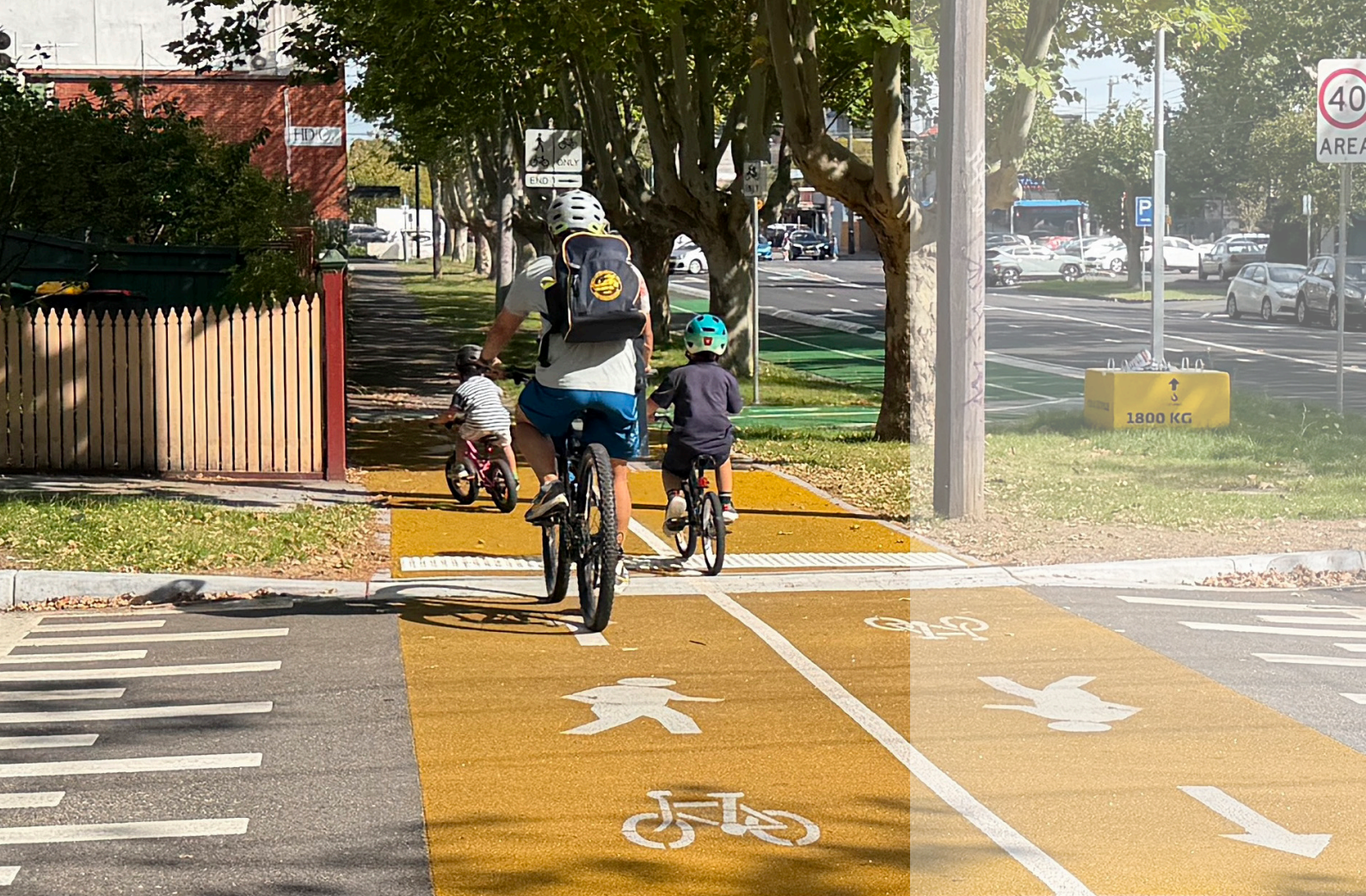
Oakleigh's new two-way cycleway on Atkinson Street.
